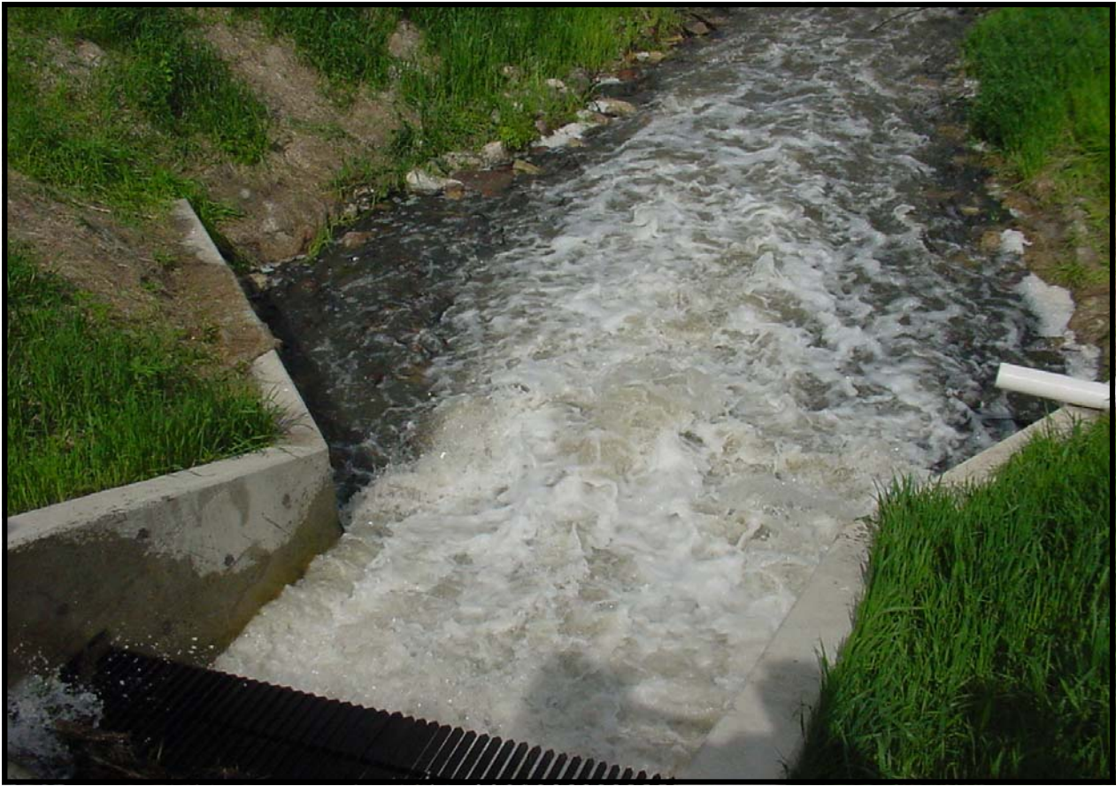
Geneva Lake ~ New fish barrier in action ~ Note the carp stacked up in the ditch just downstream of the screen. This fish barrier was installed to keep carp from entering Geneva Lake.
